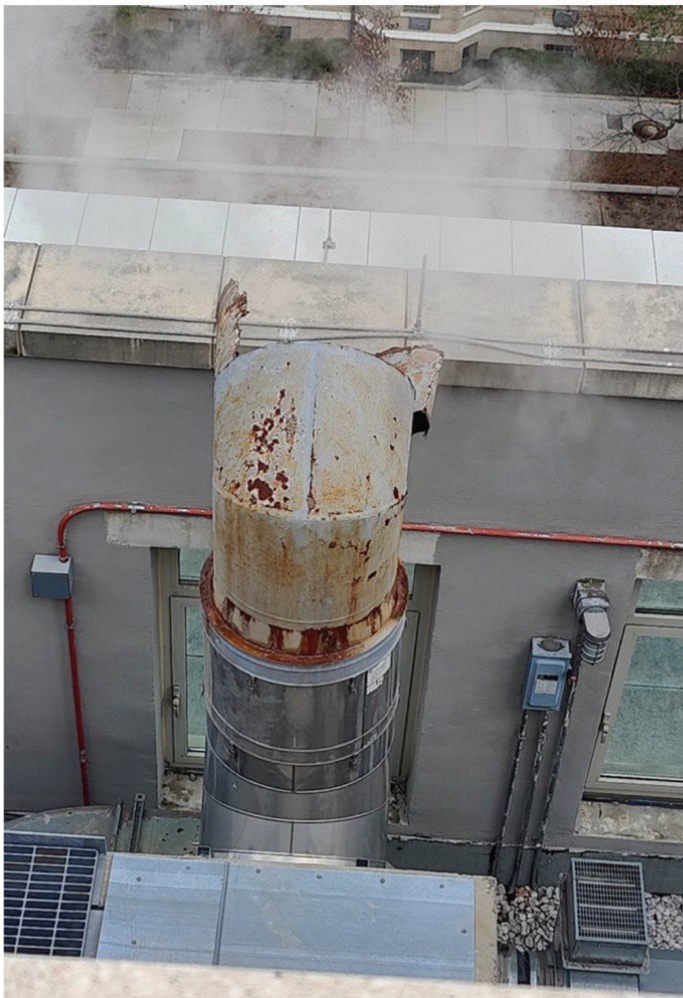
Fig 5: Evidence of corrosion
