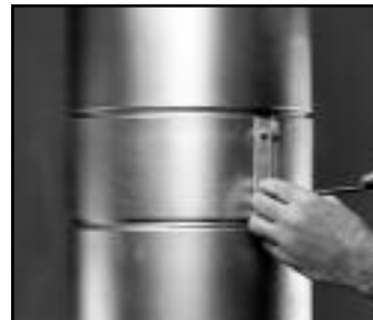
Step 4 Position Outer Channel Band around outer casing. Align with pipe grooves and tighten.
