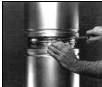
Step 3 Mate flanges of two pipes. Position Inner VB over both flanges and tighten.
